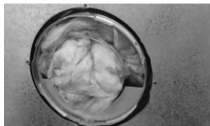
Step 5: Bend tabs out on round flue cover. Secure the round flue cover (provided) to the wrapper over the rear venting outlet. Use two (2) 3/4" long sheet metal screws
