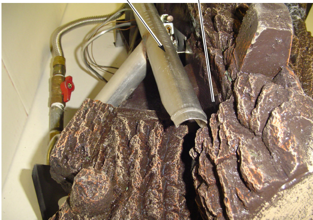
Figure 22A - Installing Middle Split Log Rear Top Side View
