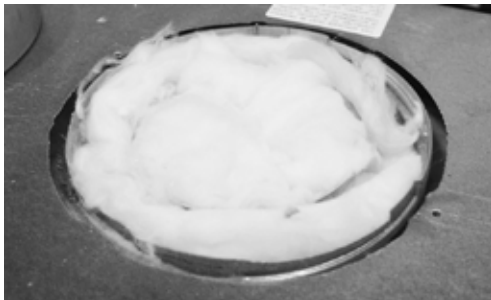
Step 3: Remove insulation from inside flue pipe.
